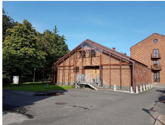
Fig. 1. The studied building located in Sege Park in Malmö, with the added glazing visible on the south and east façade. The inlet pipe to the added concrete duct for the cooling of the cavity can be seen on the left part of the picture.
