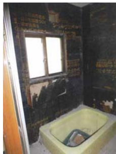
Figure 3. Removal of inner finishing tile
