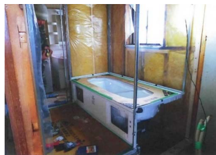
Figure 4. Setting of new bathtub
