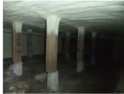
Figure 6. Insulation of undersurface of floor.
